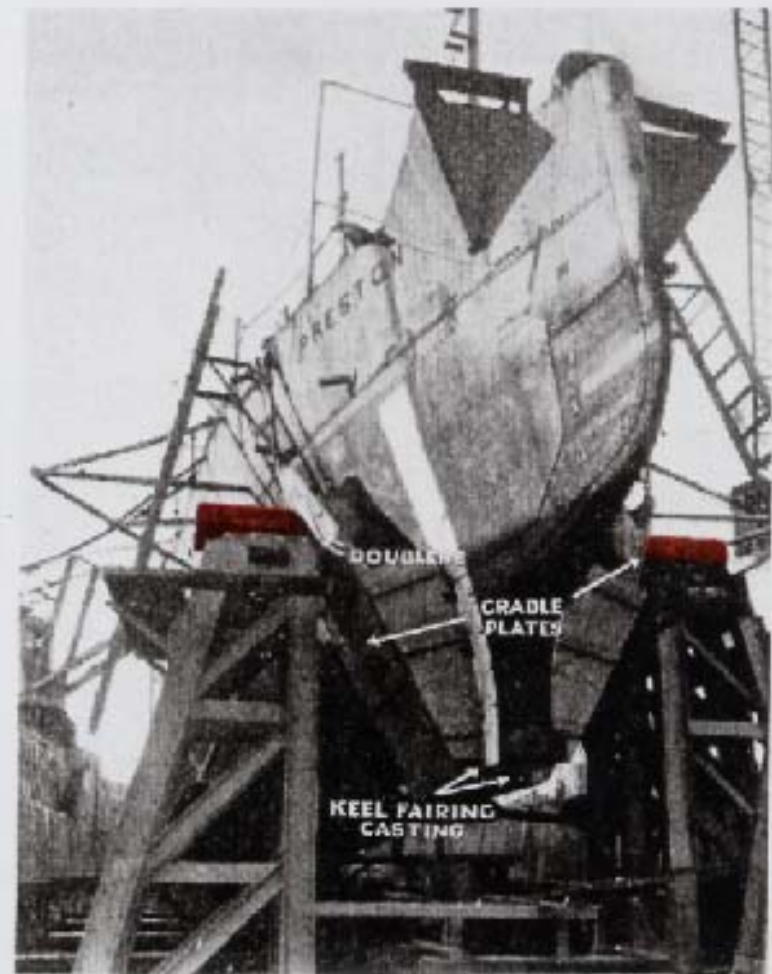
FIG. 8.—SAGGING TEST. Quarter view, showing after tower offset between cradle and hull bottom fairing casting, etc.
